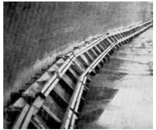
(Right) After sandblasting, wood forms were built. A very long potlife liquid epoxy bonding agent was sprayed onto concrete and steel, and a 6-1/2 sack portland cement concrete poured.
