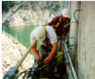
Pacoima Dam injection
