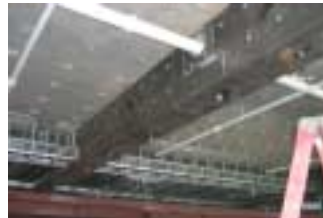
SFO beam repair
