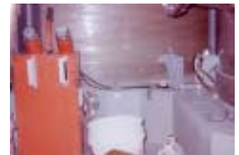
Tank bottom grouting
