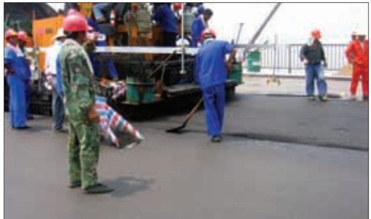
been used successfully on the Second Nanjing Bridge. The specifications required the pavement be installed in two lifts to assure that the specified 3% minimum void content was achieved or bettered. Very low void content is important to maximise fatigue resistance and waterproofing.
