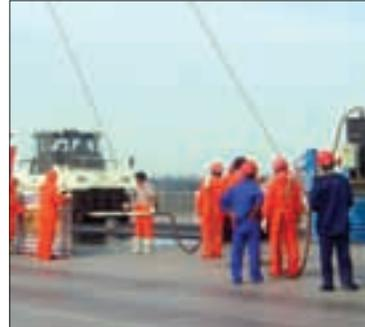
For each truckload technicians at the batch plant prepared a time sheet that informed the contractor of the maximum and minimum time that the mix should be kept in the truck. Supervisors on the deck used these time sheets to decide when that truckload should be discharged into the paving machine.
